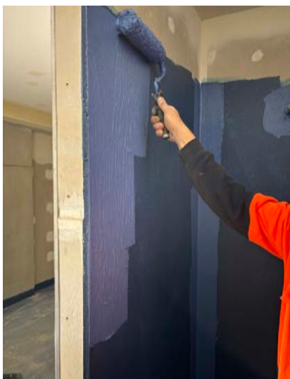
SikaTile®-111 changes colour once fully dry. It is blue when wet and turns into navy blue when dry.
