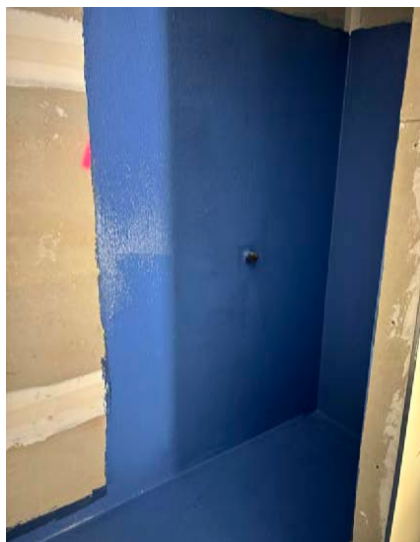
SikaTile®-111 changes colour once fully dry. It is blue when wet and turns into navy blue when dry.
