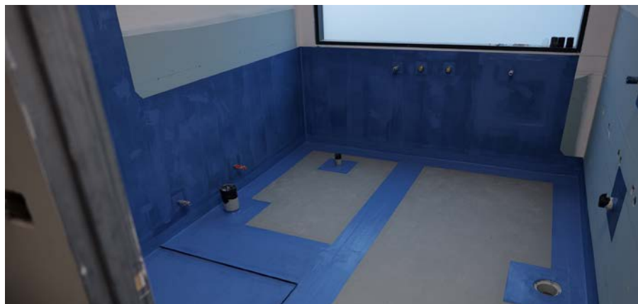
Gripset XpressLay in use for a bathroom project
