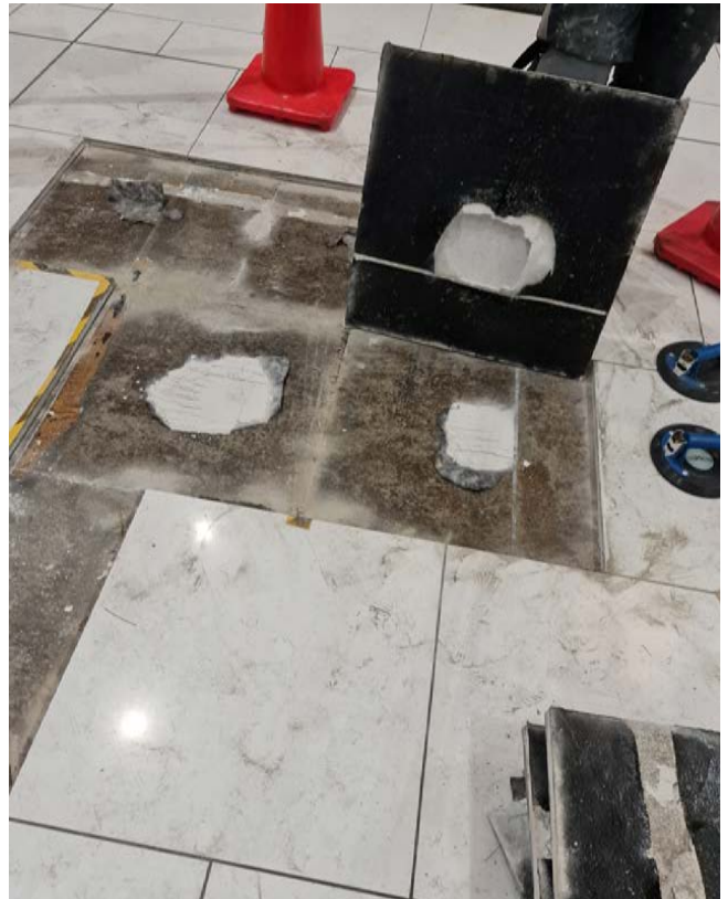
Photograph 4: Engineered stone tile installed on a crack suppression mat that curled and partially delaminated
