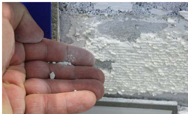
Photograph 6 shows adhesive crumbling into a powder
