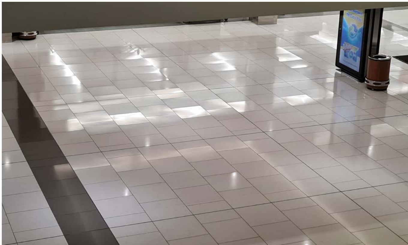
Photograph 3: Stone tile flooring which has cupped and curled in a commercial shopping centre
