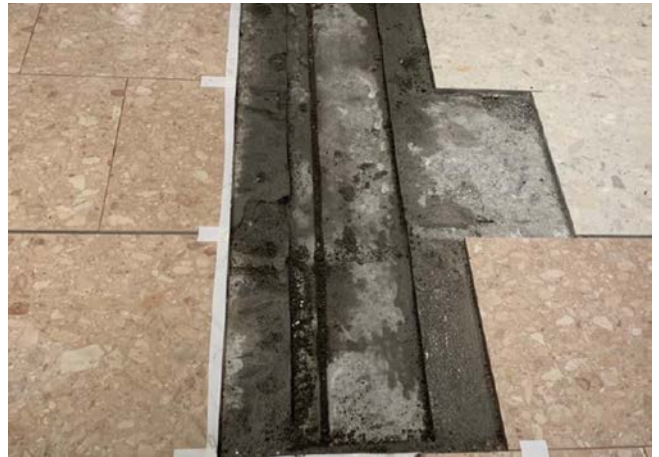
Photograph 2: Commercial shopping centre slab joint where crack isolation system failed to prevent cracking where the architect specified joints in tiles were not required
