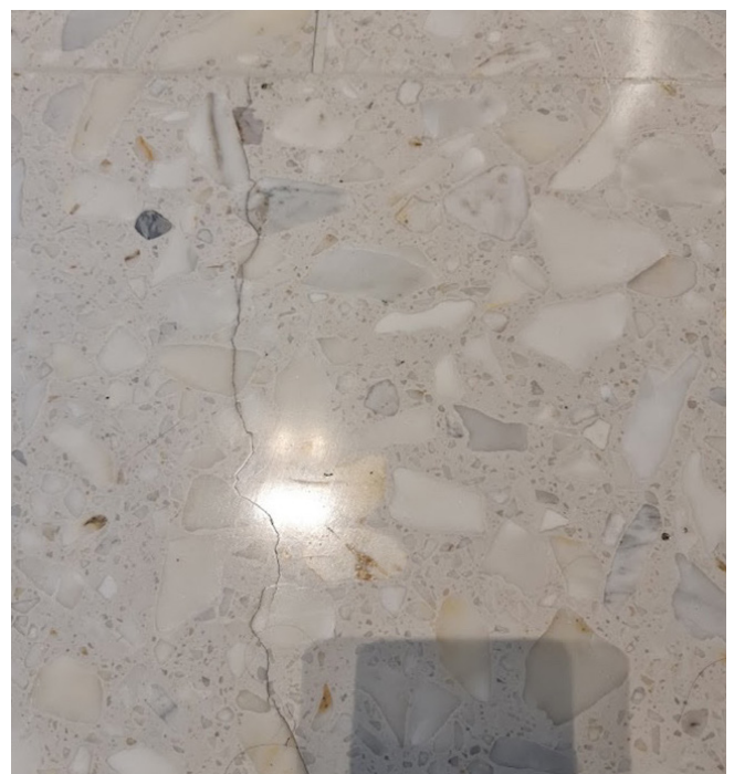
Photograph 1: Commercial shopping centre cracking in quartz tile at a cold joint location
