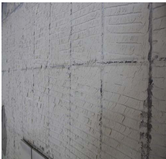
Photograph 5 shows evidence of shear forces on the tile adhesive inside a pool where failure has occurred
